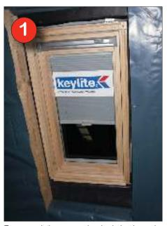
Ensure, existing vapour barrier is in place, dry and free from dust or dirt.
