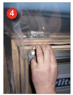
Apply inside edge of vapour collar to mastic pressing firmly. Start at top of the window and work down.
