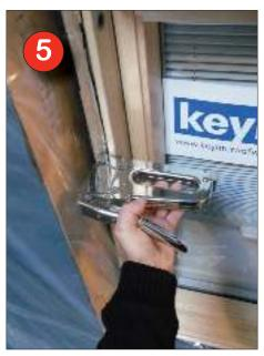
For added seal protection staple around inside edge. Ensure to staple through mastic!
