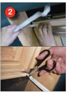
Apply mastic strips in the centre of the plasterboard groove. Trim lengths to suit.
