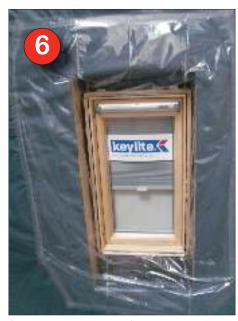
Seal the outside edges of the vapour collar to the existing vapour barrier with tape provided.
